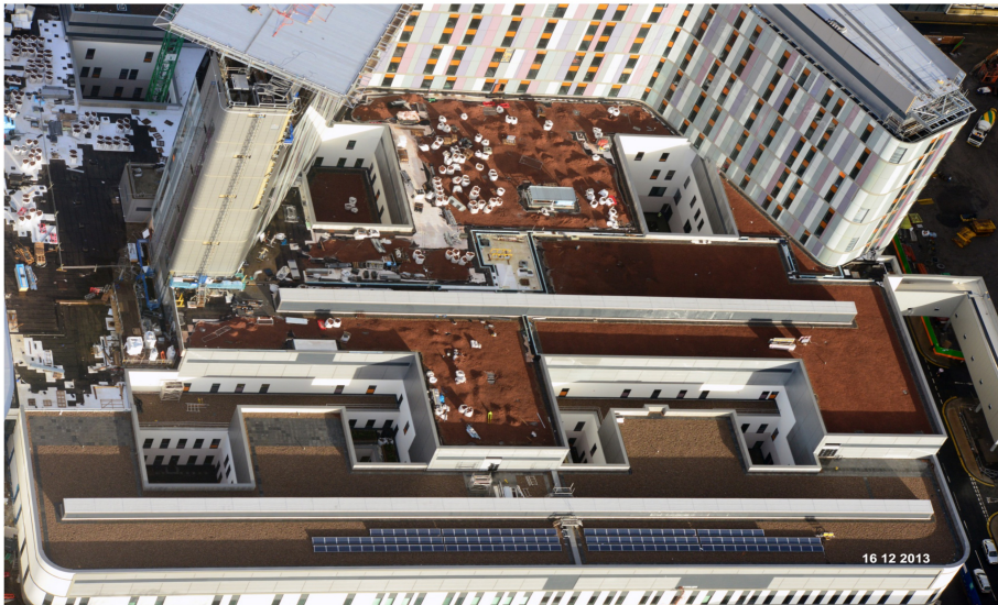
Solar Panel Installation
